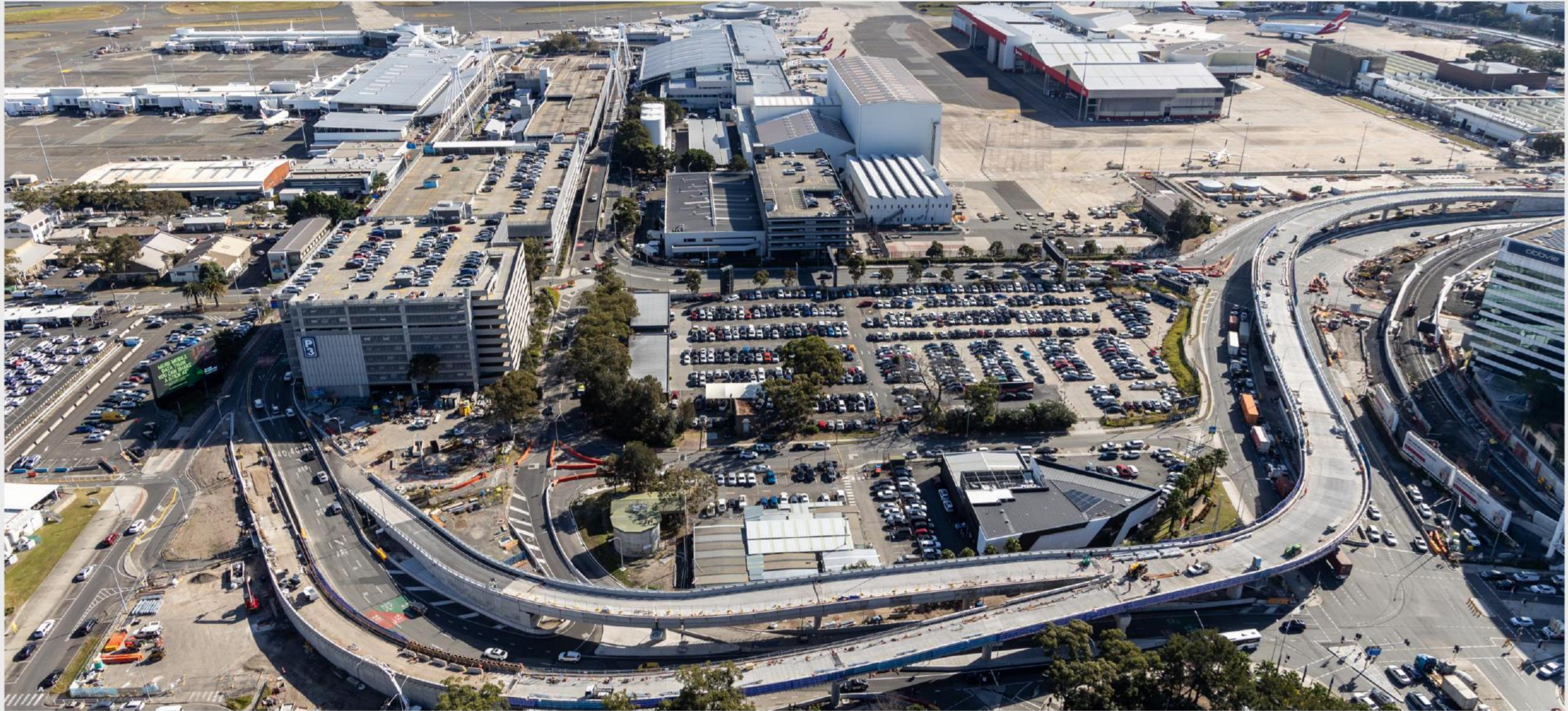
Flyover – Entry to Domestic Terminals
