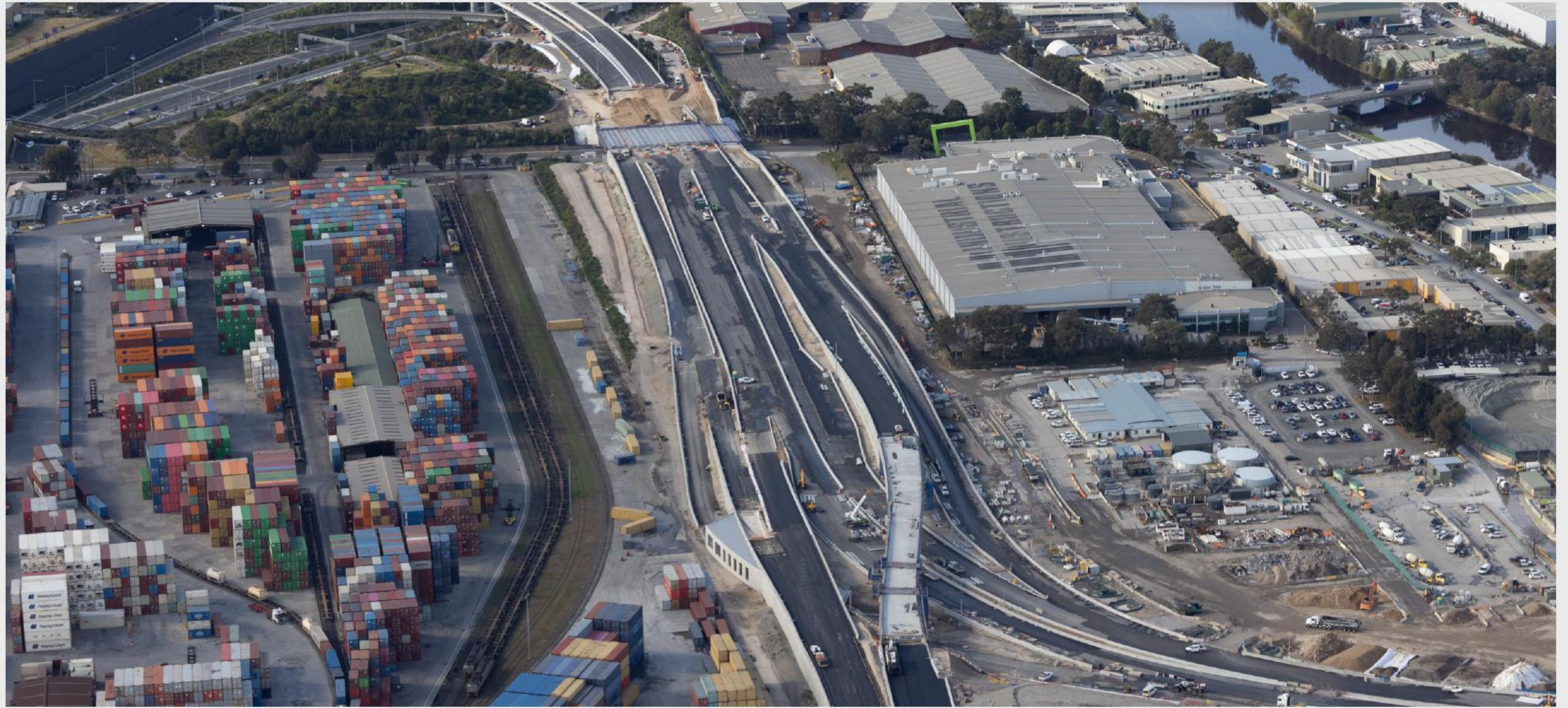
Northern Lands – crossing Canal Rd
