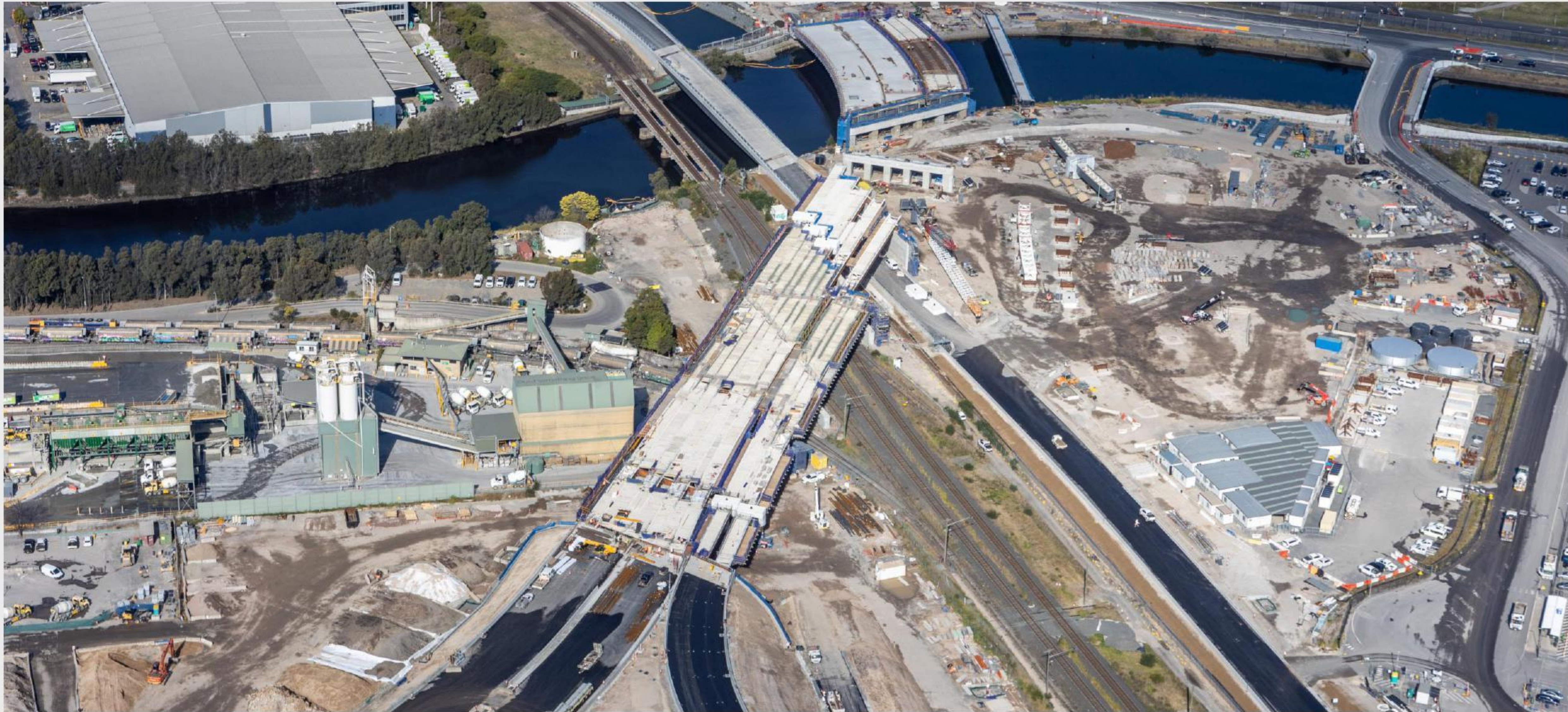
Alexandra Canal – Bridge works between Qantas Drive and St Peters Interchange
