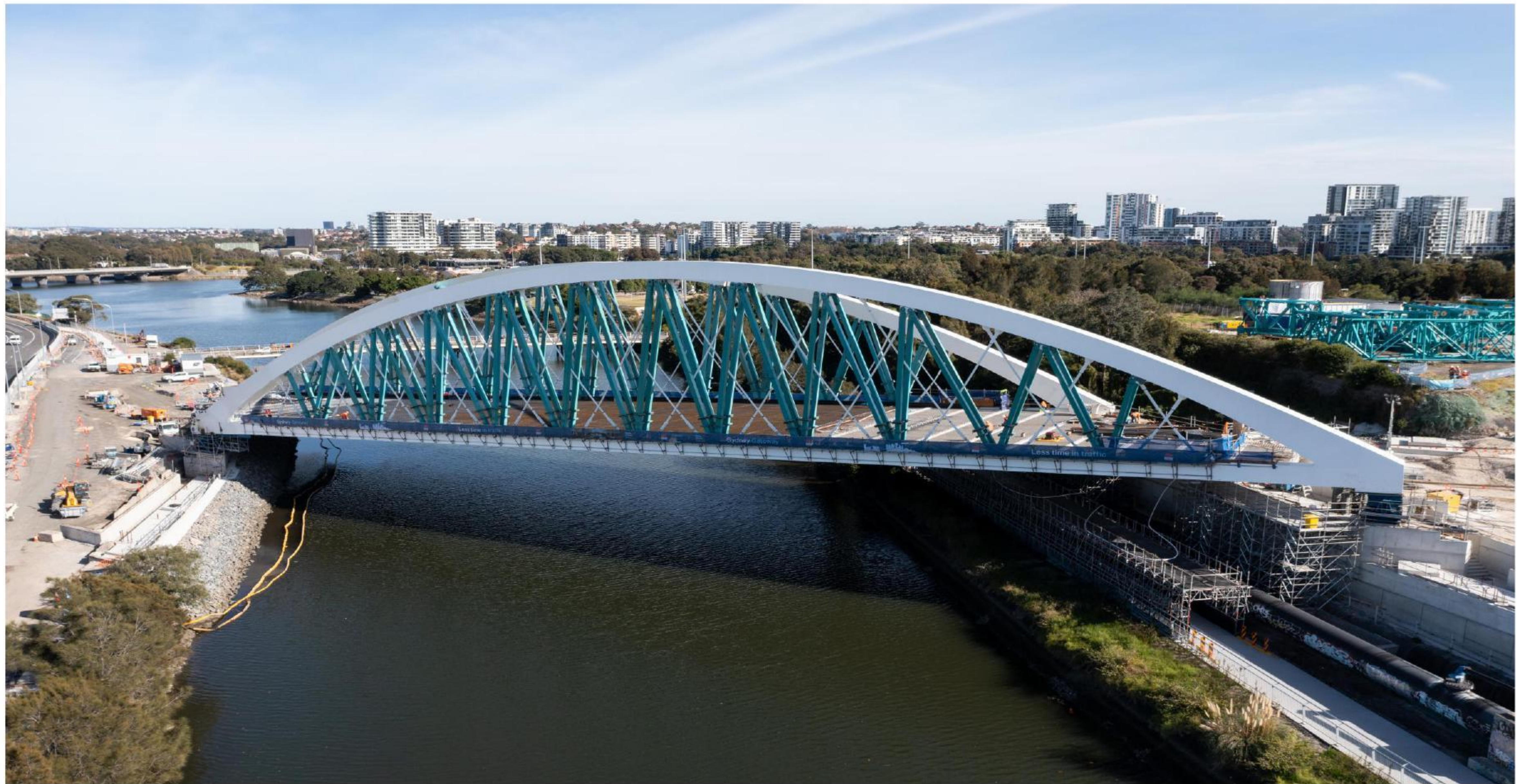
Tempe – Bridge launched over Alexandra Canal
